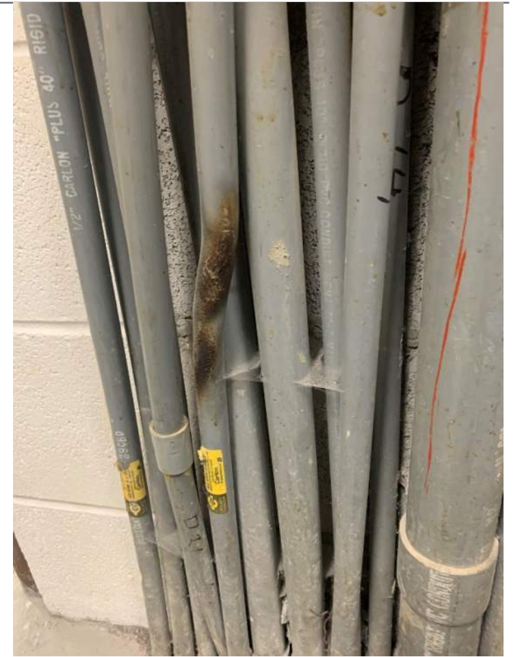
E5: Conduit shows signs of electrical fire and should be replaced.
