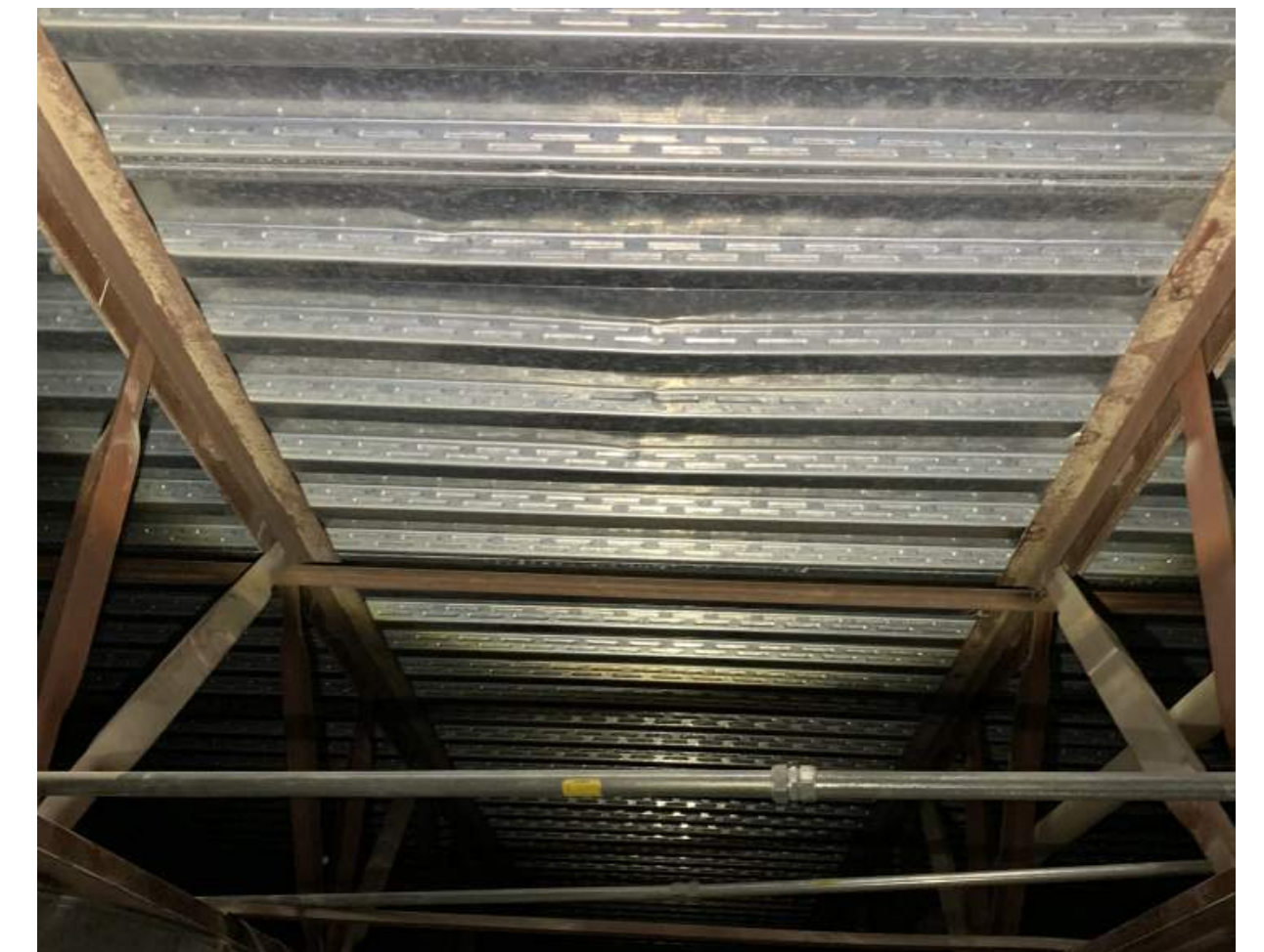
Figure 6. Deformed Metal Deck Below Weight Room (1985 Addition)
